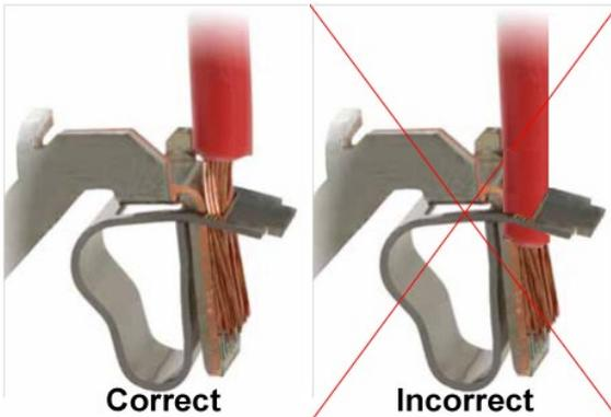
4. Remove the screwdriver. The clamp pressure will keep the wire in place. No exposed wire should protrude past the cage opening
