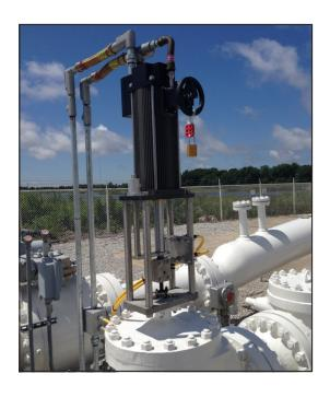
directly to a linear force. This unique design provides high force and fast response needed for the application, as well as long life to minimize maintenance. Controls for the actuator were provided by Rockwell Automation, seamlessly integrating the Exlar valve actuator into the overall pump station control. The control scheme also includes continuous diagnostic capabilities; providing information on the health of the valve as well as the actuator
